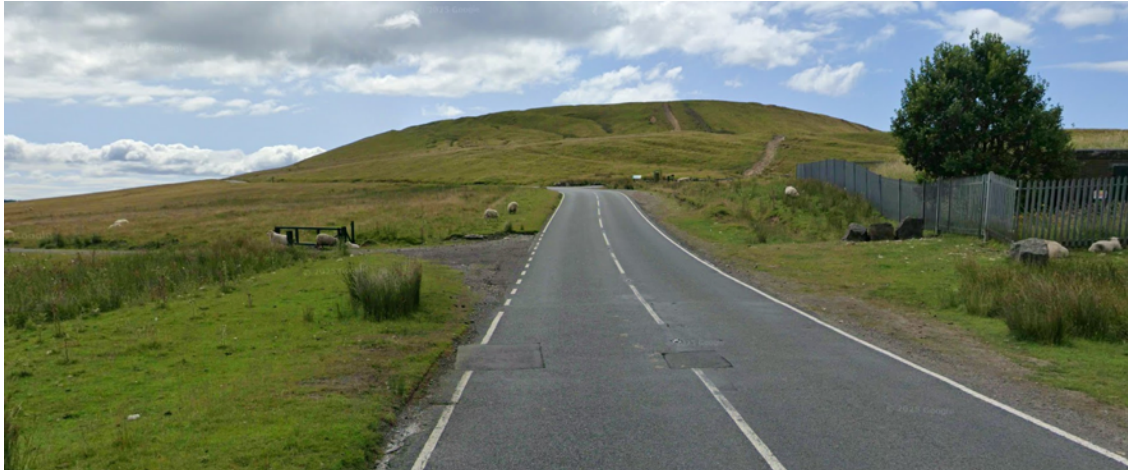
Figure 3 Site Access Junction (Viewed from the North)
